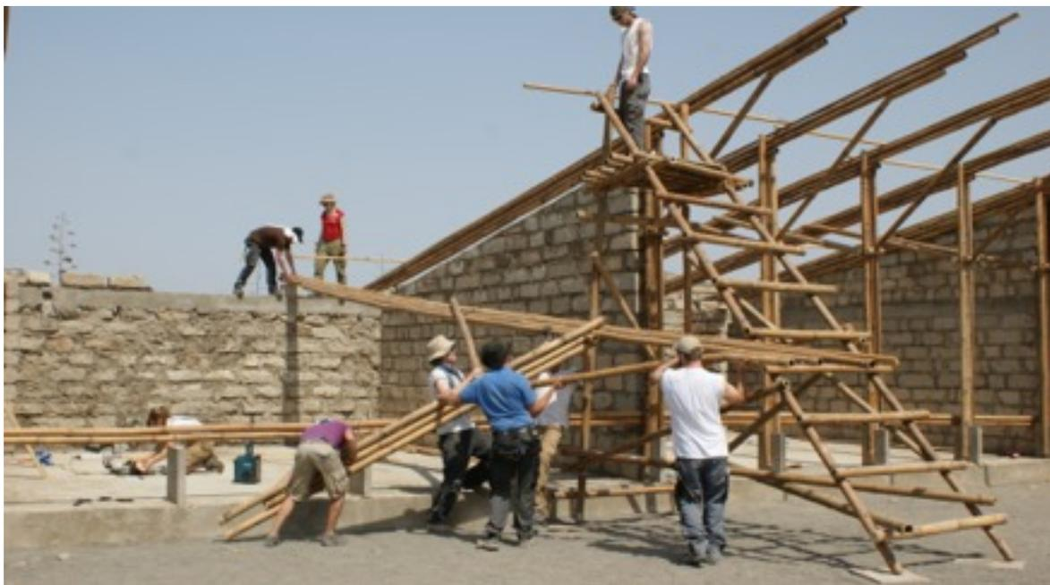
*fig. 9 Assembling of the roof structure of the workshop building*
